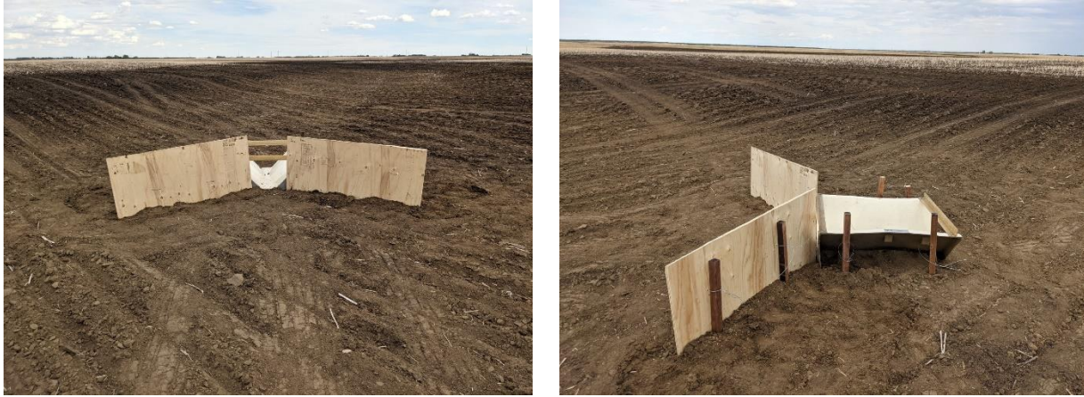
Figure 5. Example of H-flume installed at the exit point of the surface ditch from each basin.
