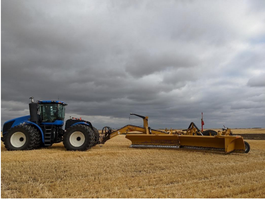
Figure 2. Field equipment used for construction of surface ditches.
